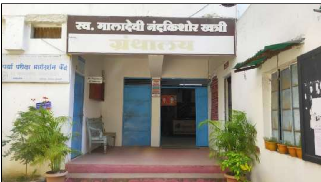
Front View of Library
